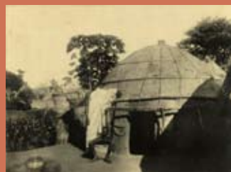
Cupola construction of a house in Wukari which will still be covered by a conical thatch roof
